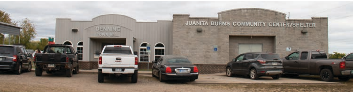
With help from federal and state grants and loans, Denning has been able to build a new town hall and attached community center/tornado shelter. The town has also built a new public works building to replace the destroyed water department.
