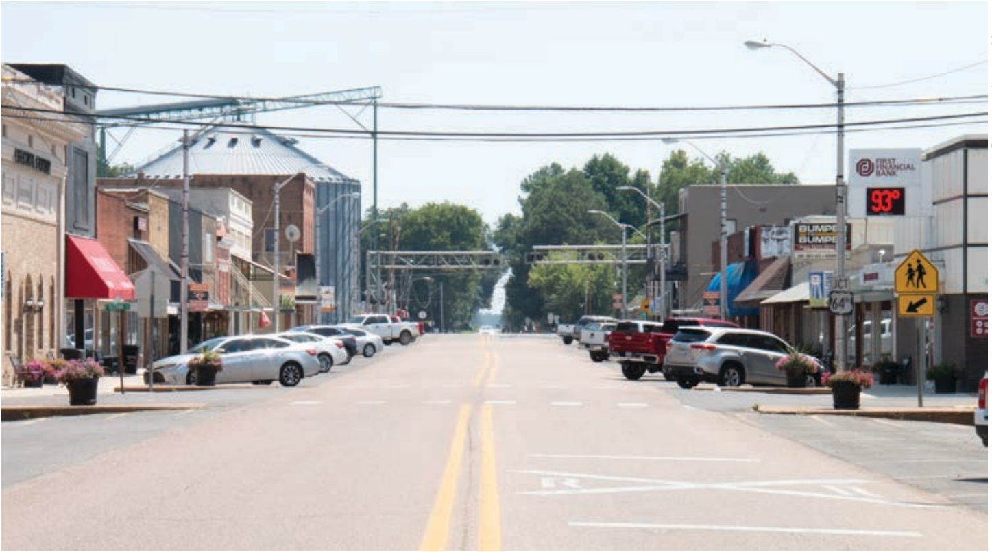
Granaries loom behind the McCrory Commercial Historic District, which is listed on the National Register of Historic Places.
