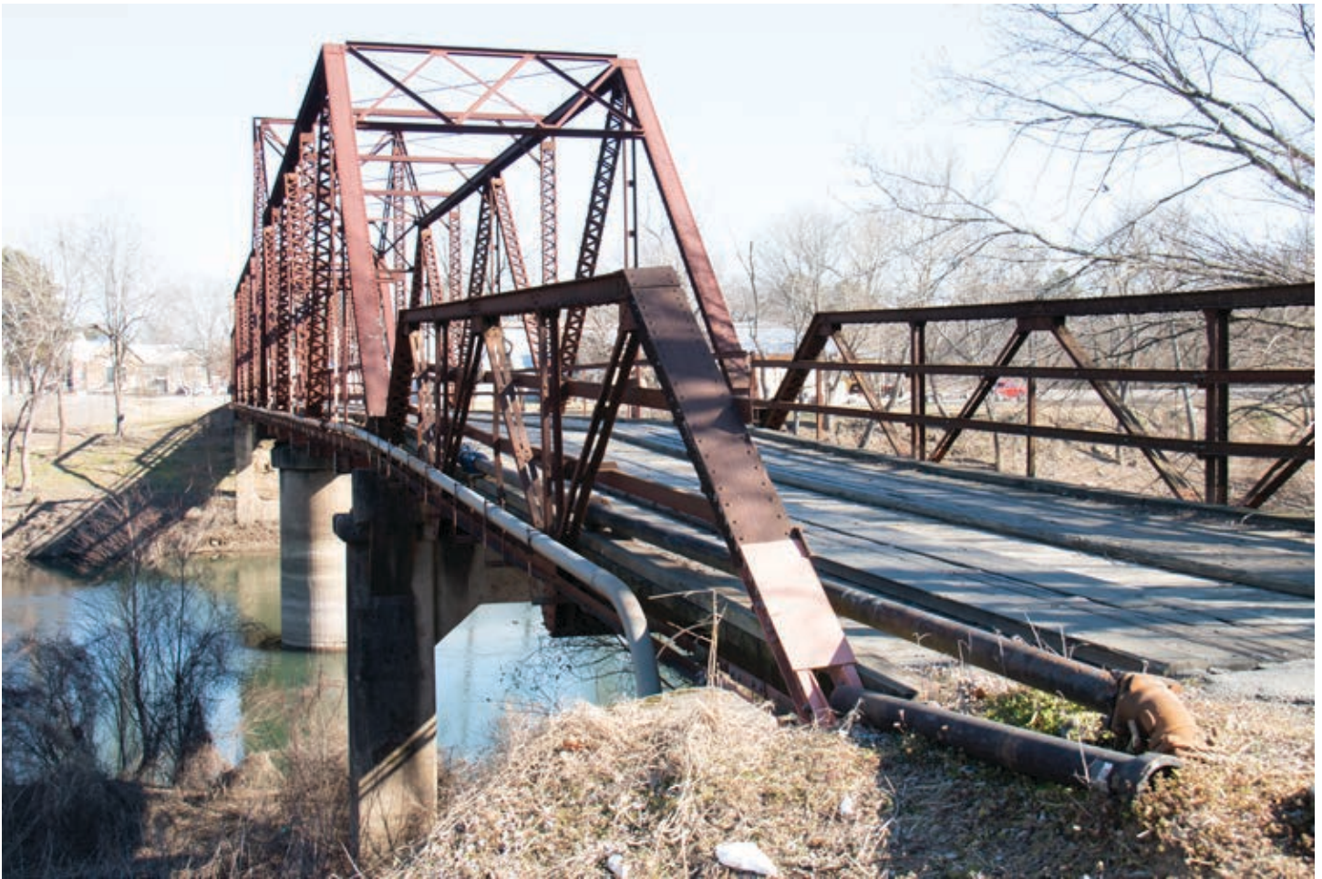
The single-lane, cantilever swing bridge over the Little Red River in Judsonia was built in 1924 and was essential to the city's early development. It was listed on the National Register of Historic Places in 1990.
