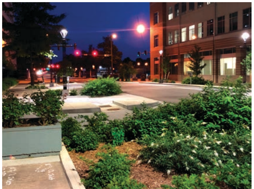
The bioswales that line Main Street in downtown Little Rock collect and filter stormwater runoff, limiting the pollutants that enter the storm drains.
