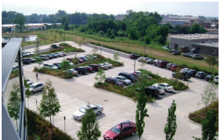
The grounds of Heifer International’s Little Rock headquarters feature numerous runoff-controlling, low-impact design features, including retention ponds, bioswales and porous parking spaces.
