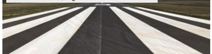
The overlay provides a smooth runway and restores the dark, high-contrast surface color.
