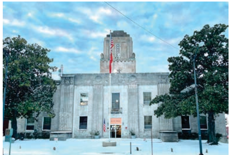
City Clerk Heather McVay snapped this photo of El Dorado City Hall during a walk to experience the winter weather. According to the National Weather Service in Little Rock, El Dorado received 10-14 inches of snow from February 14-18.
