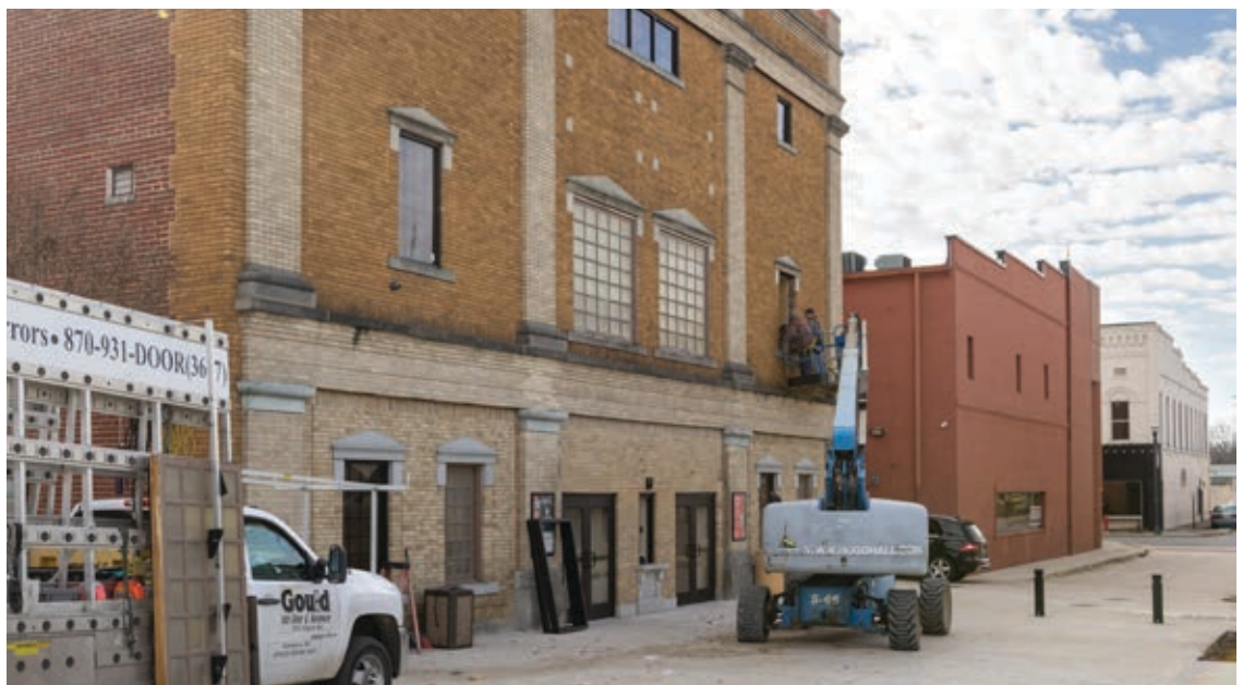
The circa-1926 theater received upgrades both inside and out, including new window frames and windows.
