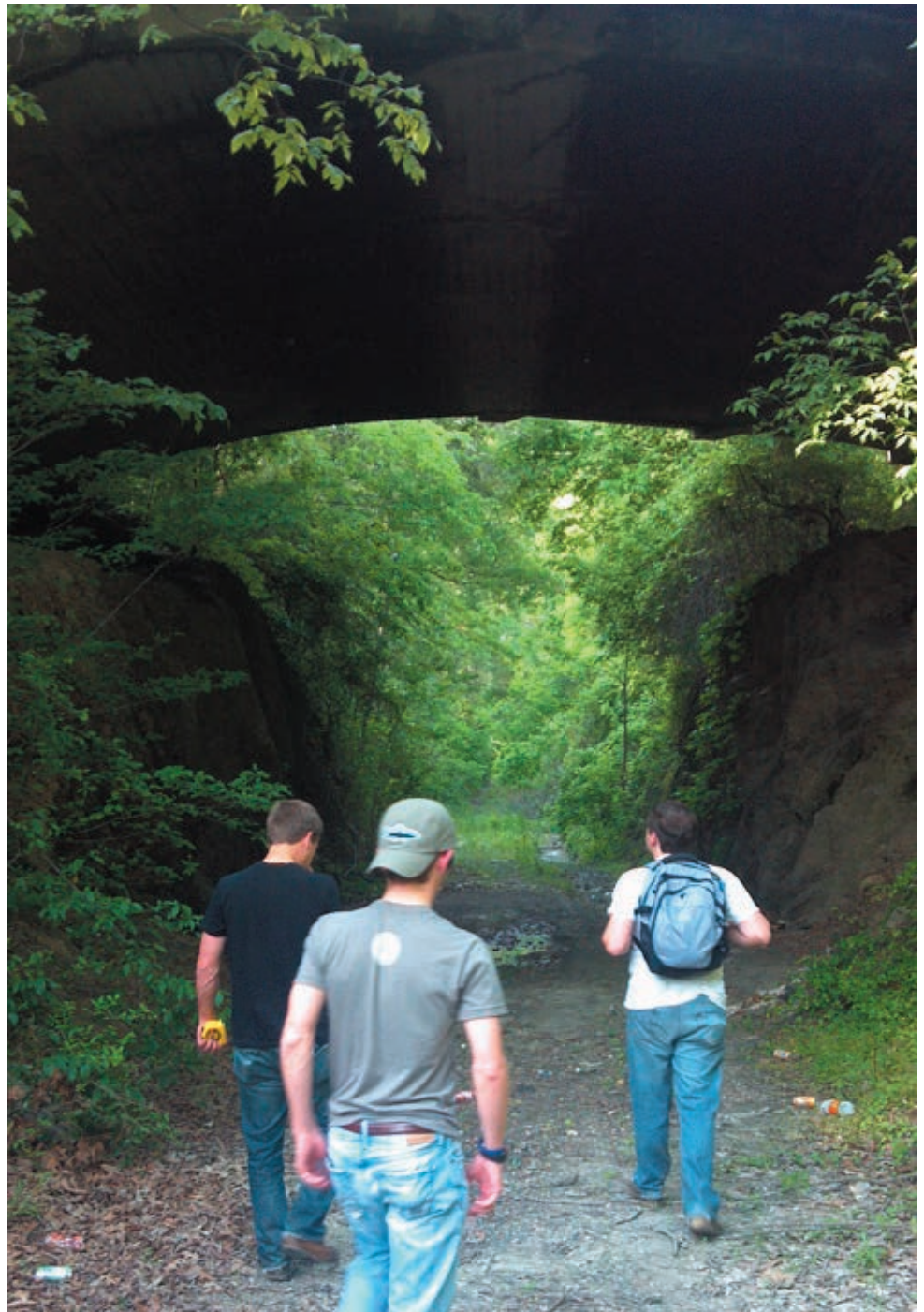
A team explores what will become the route for the ambitious Southwest Trail connecting Little Rock and Hot Springs.
