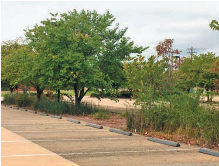
Forest-friendly development can include the use of flush curbs that allow rainwater to be directed toward areas where trees grow.
