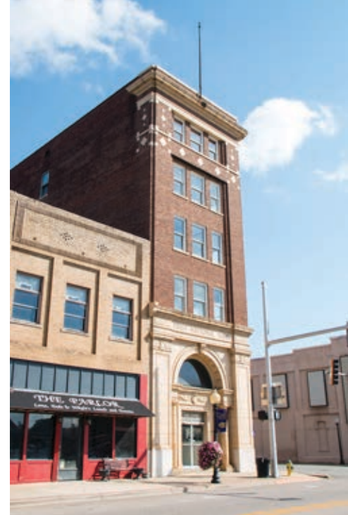
One of downtown's unique features is the old First National Bank building, the tallest office building between Little Rock and Fort Smith. It is listed on the National Register of Historic Places.
