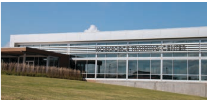
The new state-of-the-art Workforce Education Center at the UofA Community College at Morrilton opened in April of this year.
