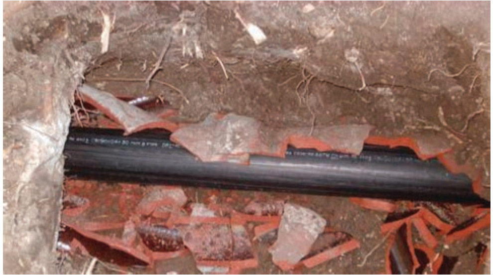
Example of pipe bursting.
