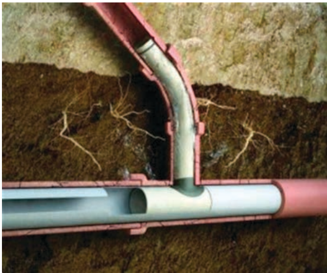
Example of internal service connection and relining.
