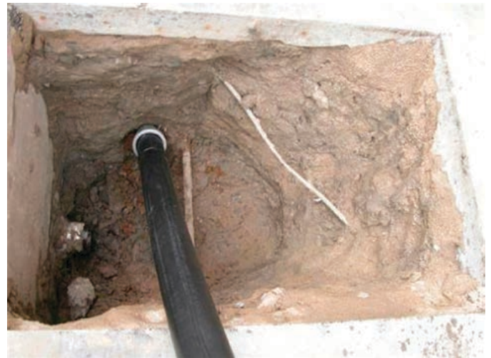
Example of sliplining.
