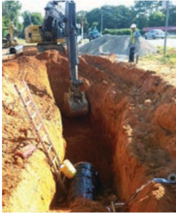
Workers install a 24-inch water main in Benton.
