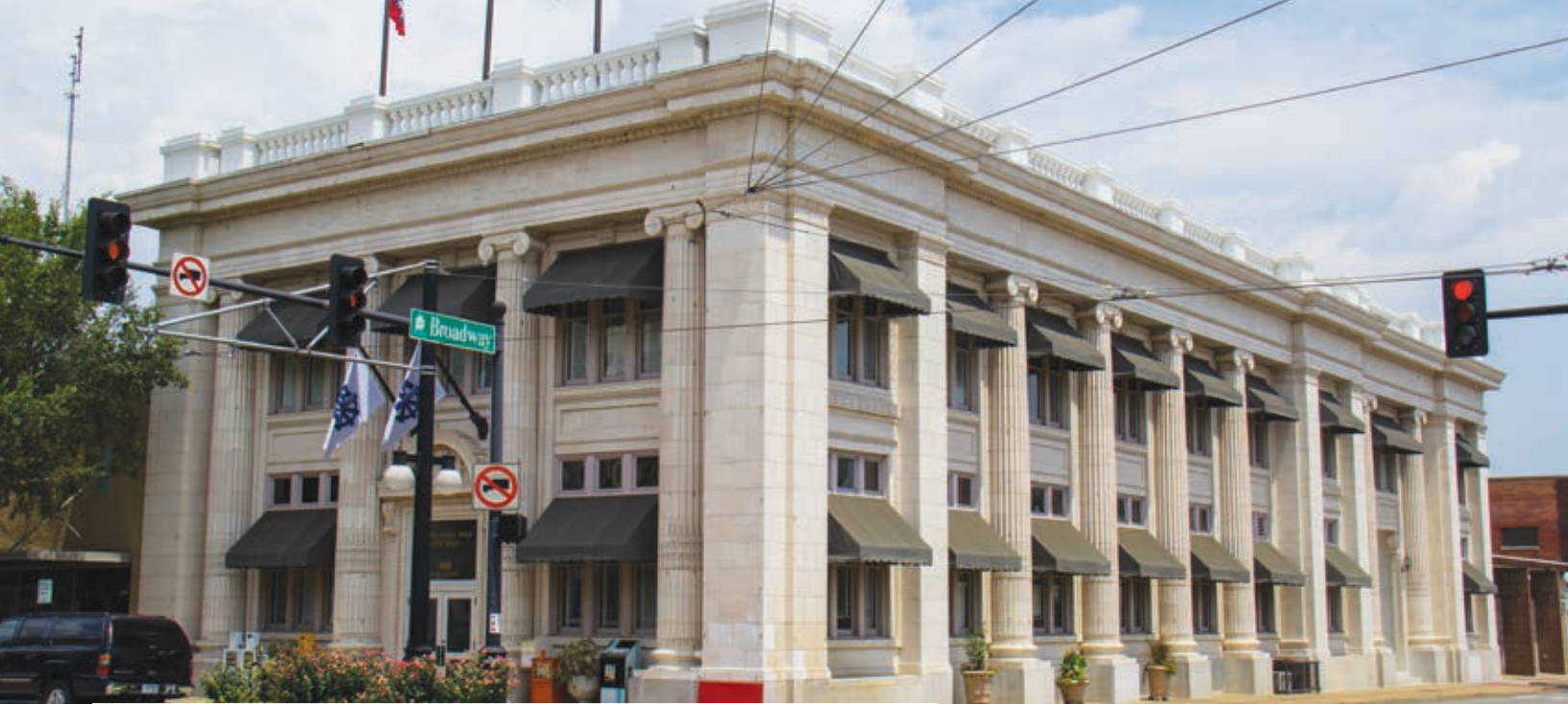
North Little Rock City Hall's exterior is made of cast stone and terra cotta block.
