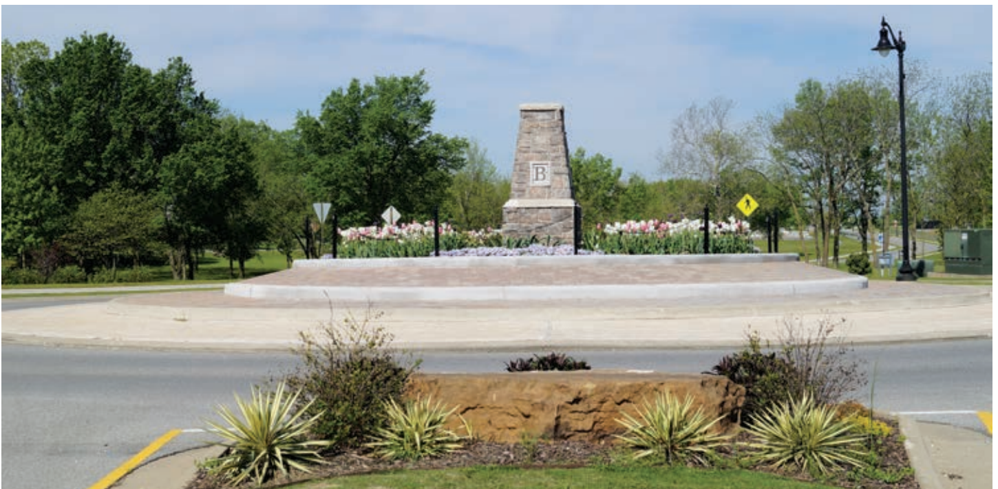
Bentonville's Memorial Park area features an aesthetically pleasing, traffic calming roundabout. A concrete and paver apron allows for large truck traffic to navigate the intersection when necessary.
