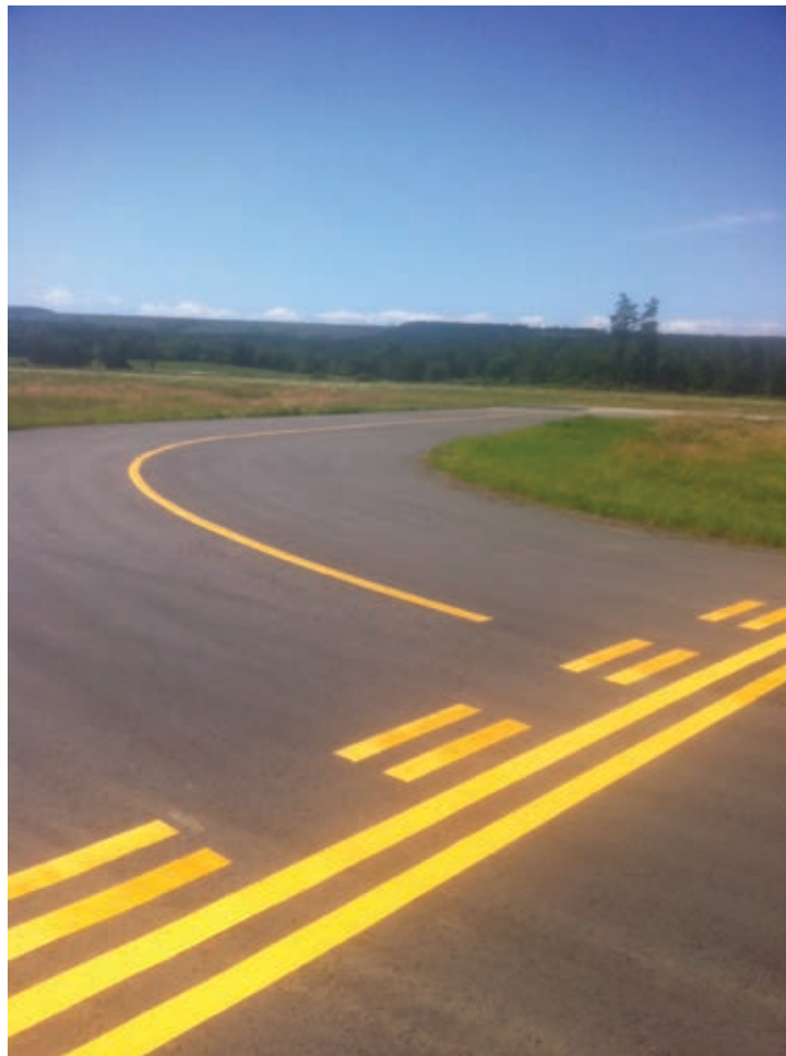
Waldron Municipal Airport used a phased funding approach for its parallel taxiway project. Phases I-III—design, wetland mitigation, and taxiway construction—are complete. Phase IV, lighting installation, is in progress.
