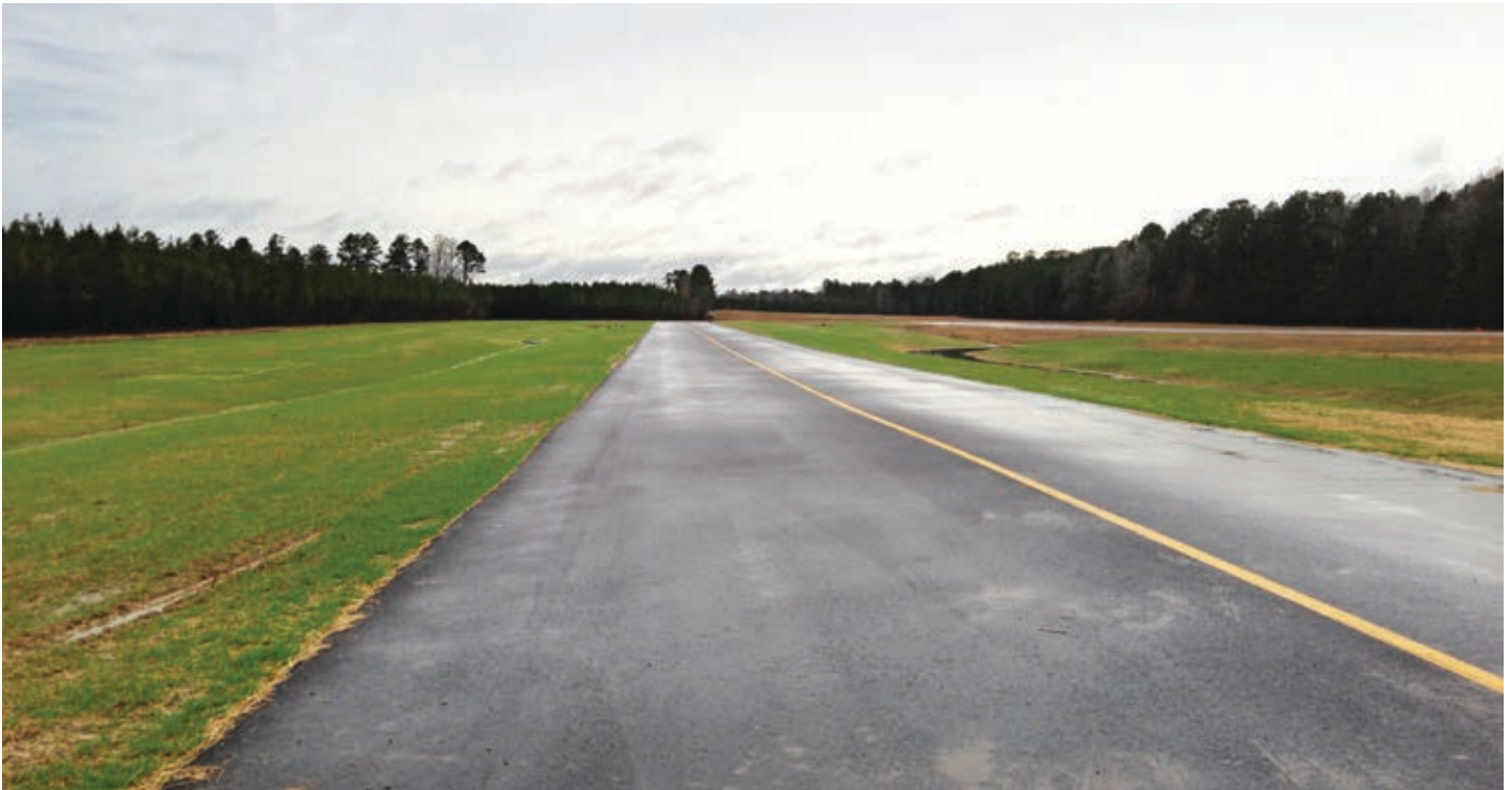
The recently completed parallel taxiway at Warren Municipal Airport cost $689,576 and received federal grant and discretionary funding, as well as state grant funding.
