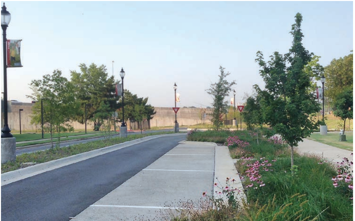
New developments at Little Rock's MacArthur Park include rain gardens, shade trees, and pervious concrete pavements, which add beauty while mitigating runoff.
