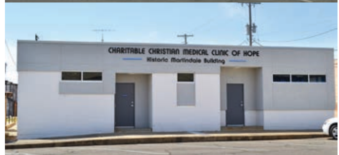
Hope's historic Martindale Clinic, before and after renovation.
