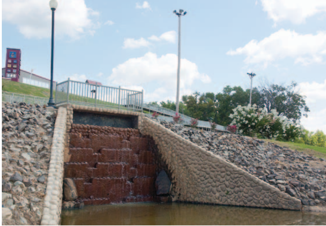
Where runoff from downtown Camden once poured from a culvert into the river, this waterfall provides an attractive drainage solution for the city’s riverfront development.
