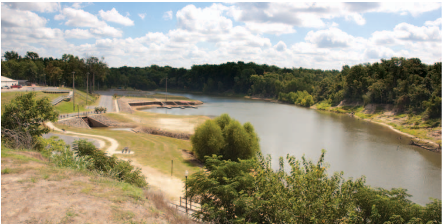
What was just a few years ago an overgrown, muddy and generally unapproachable riverfront now features recreation areas, parking, a boat ramp, boat dock, river walk, and, just out of view, an amphitheater.
