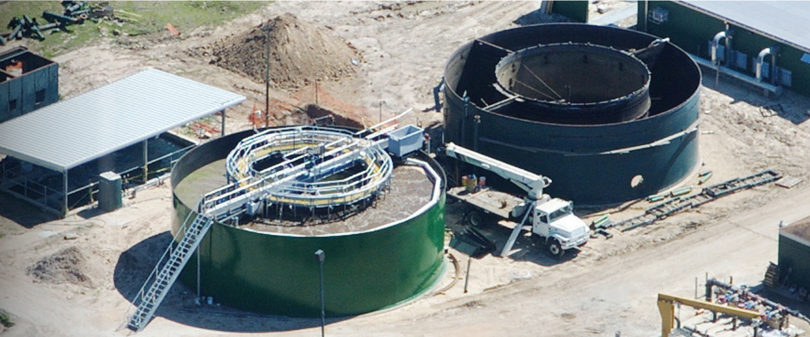
Spencer Road Municipal Utility District- WWTP Rehabilitation - Houston, Texas
