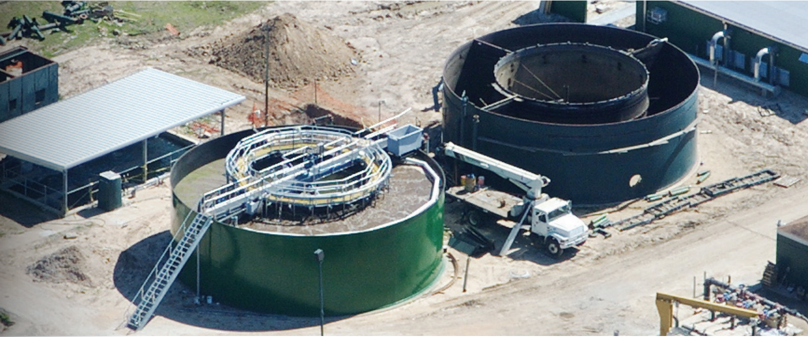
Spencer Road Municipal Utility District- WWTP Rehabilitation - Houston, Texas
