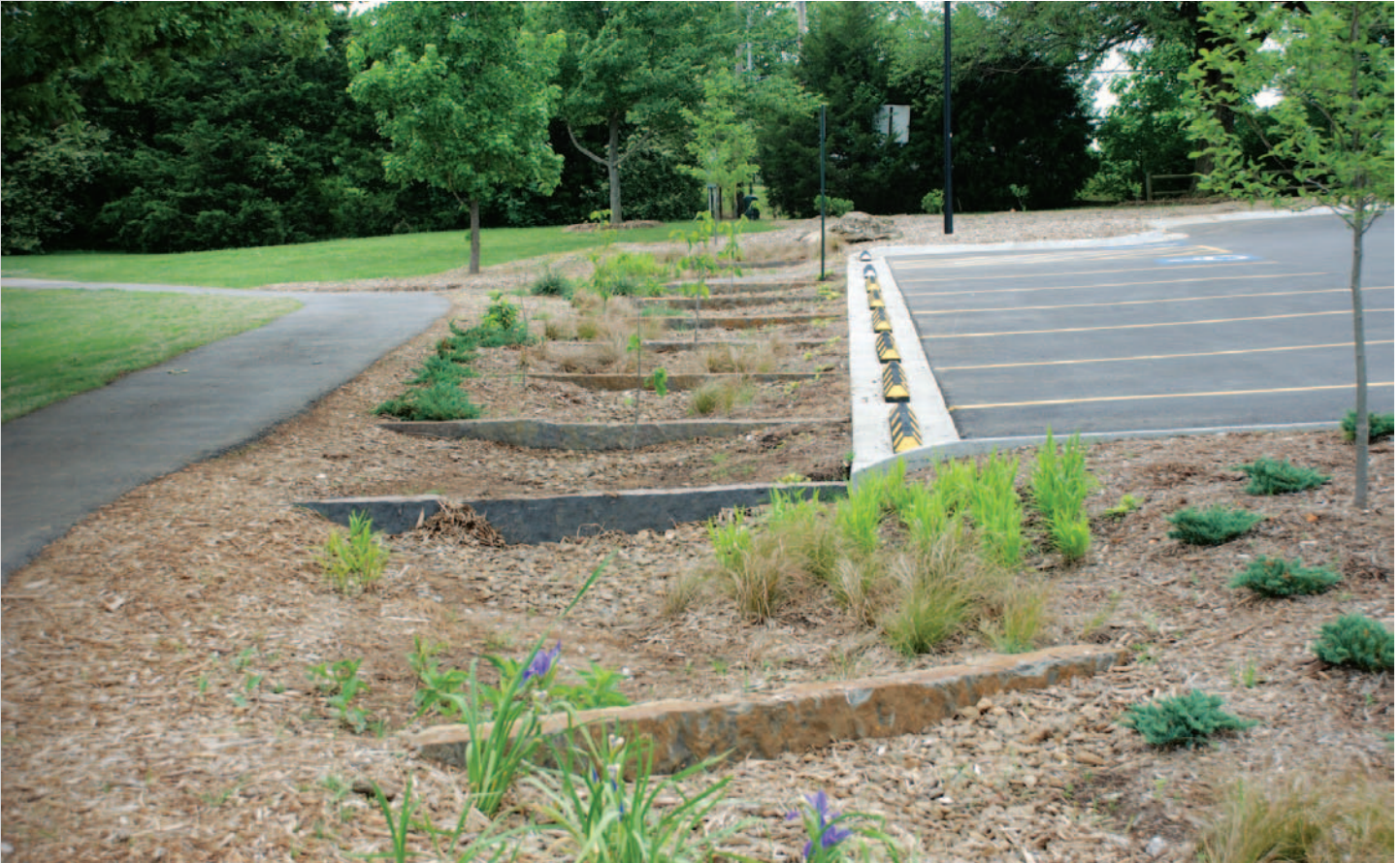
This bioswale in Fayetteville captures pollutants and reduces runoff flooding from the parking lot. The project was funded by the city's parks department and by a grant from the USDA Forest Service.
