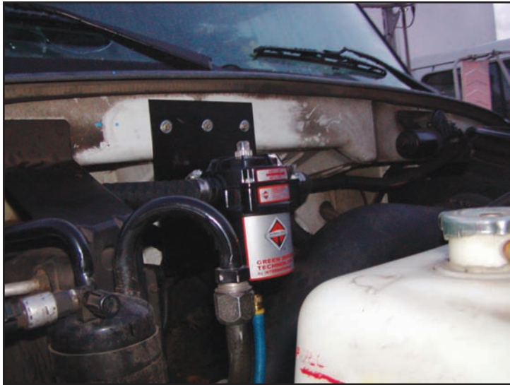
Emissions-reducing filter muffer systems on North Little Rock diesels are helping keep pollutants out of the air.
