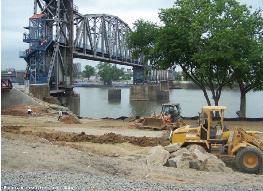
PHOTO COURTESY CITY OF LITTLE ROCK
