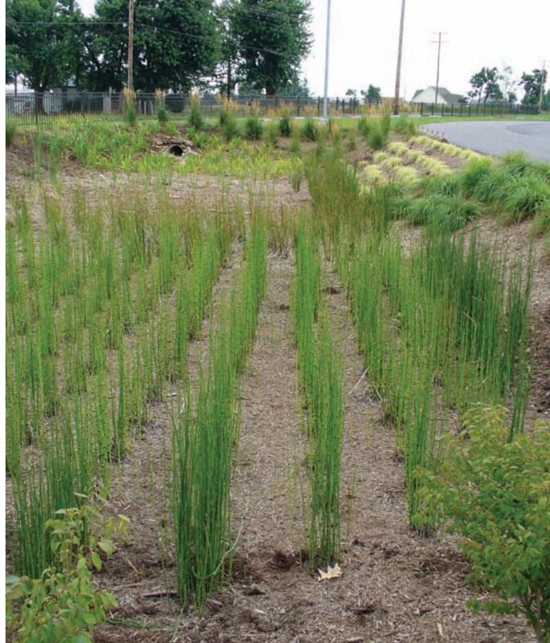
Bio-swales accommodate water filtration and absorption.
