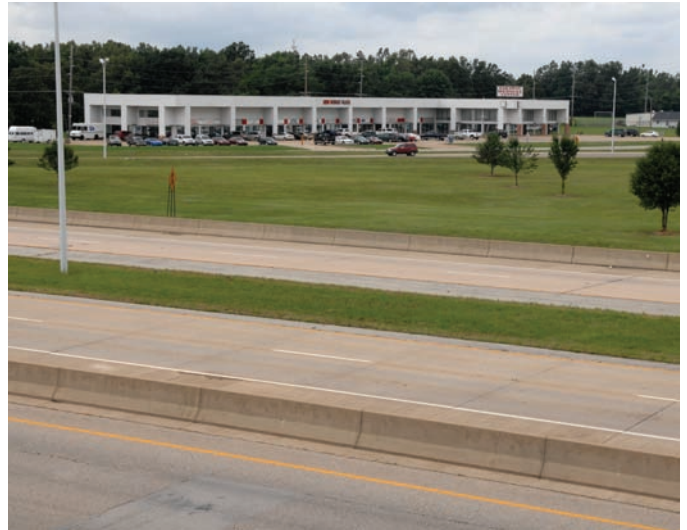
After, Caraway Road and Hwy. 63, northwest side.
